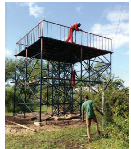
Erecting tank towers in Serengeti for the Borehole Project
